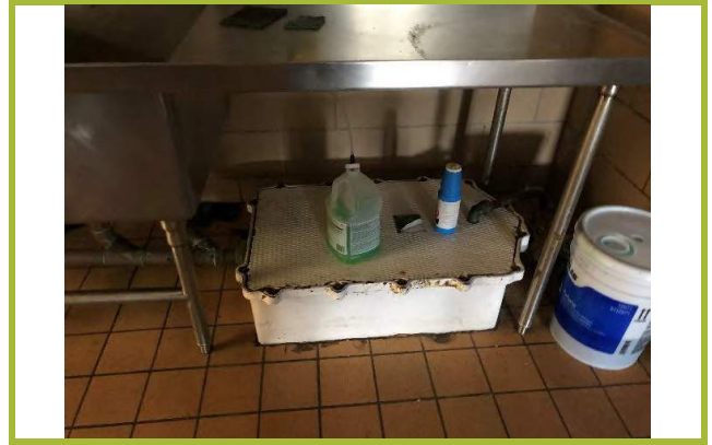
Photo #20: Grease trap.
