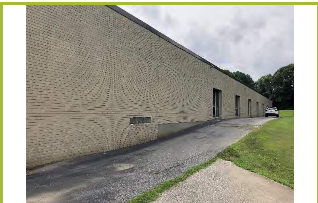
Photo #5: Western exterior of the 1969 addition.
