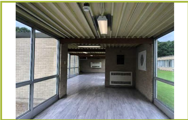
Photo #15: Southern hallway connecting the 1969 addition to the original portion of the site building.
