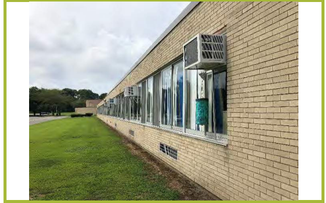
Photo #2: Eastern exterior.
