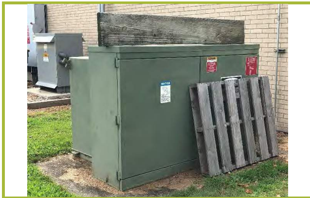
Photo #9: Transformer along the northern exterior of the site building.
