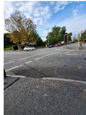
Photo 3: Eastbound Approach on Read Street
