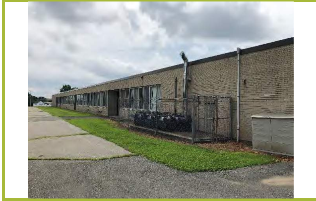
Photo #7: Northern exterior.
