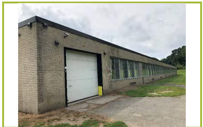
Photo #6: Western exterior of the 1965 portion of the site building.
