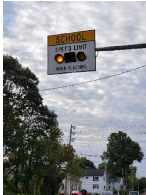
Photo 11: One of Two School Zone Speed Limit Flasher Sign
