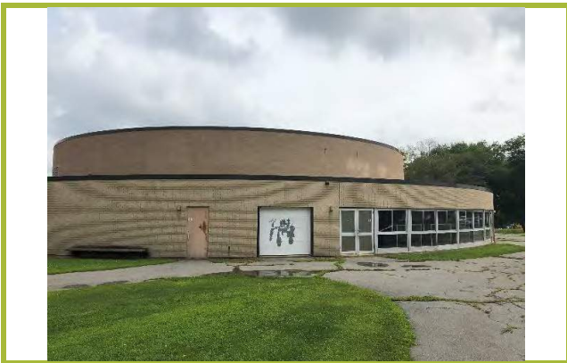
Photo #3: Southeastern portion of the site building, the school gymnasium.
