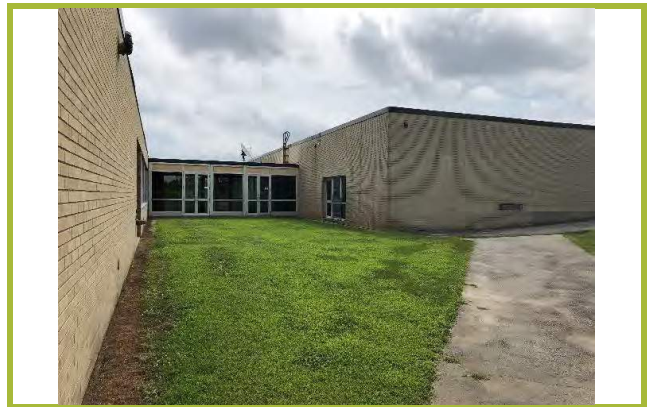
Photo #4: Connection between the 1965 and 1969 portions of the site building.
